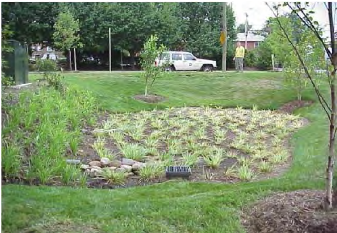
Figure 6-4: Photo of Bioretention Draining a Rooftop at a Commercial Facility (Virginia DEQ 2011c)
