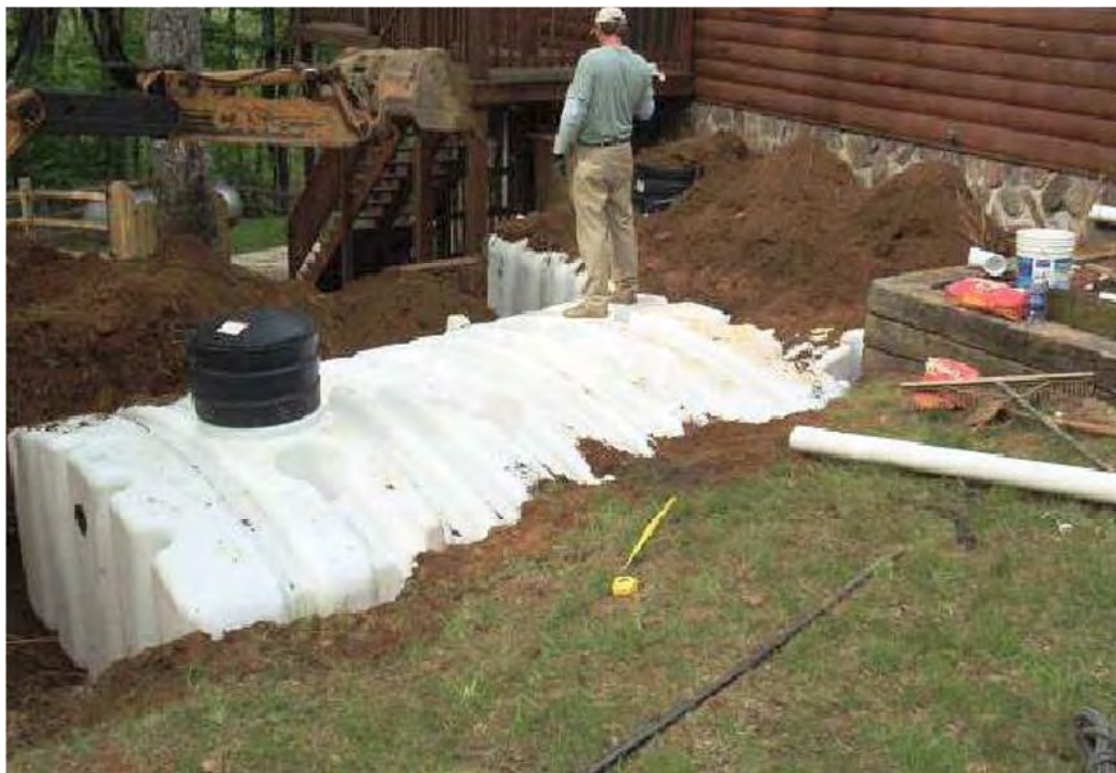
Figure 6-9: Subterranean Cistern (Virginia DEQ 2011f)
