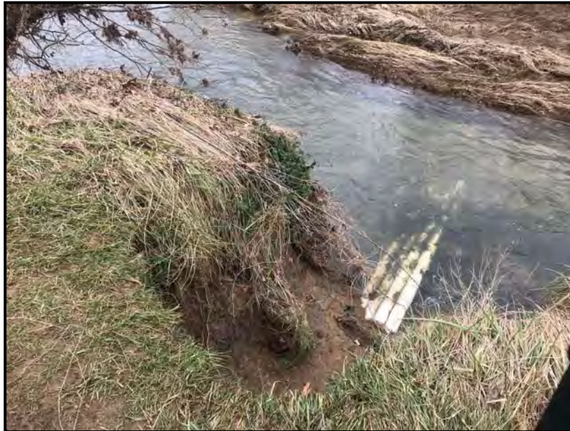
Figure 4-15: Exposed Pipe within the Stream, within Lower South Fork Catoctin Creek
