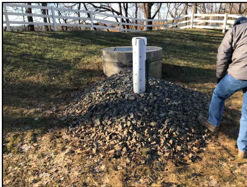
Figure 4-54: Perforated stack pipe, gravel filter, and grated outflow with low flow orifice in Dry Pond JC7170
