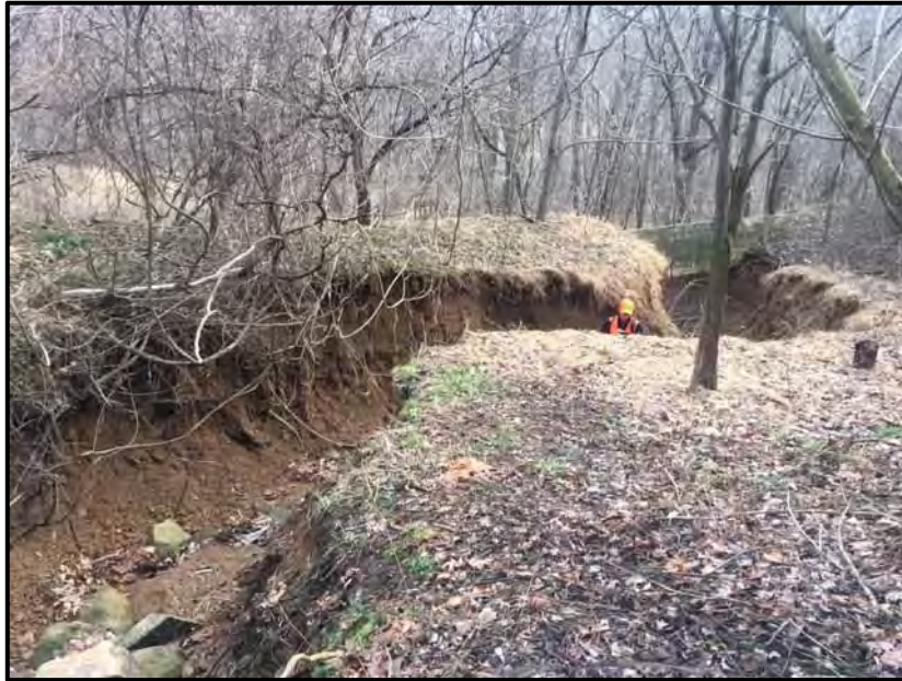
Figure 8-21: Outfall channel erosion presenting an opportunity for RSC design
