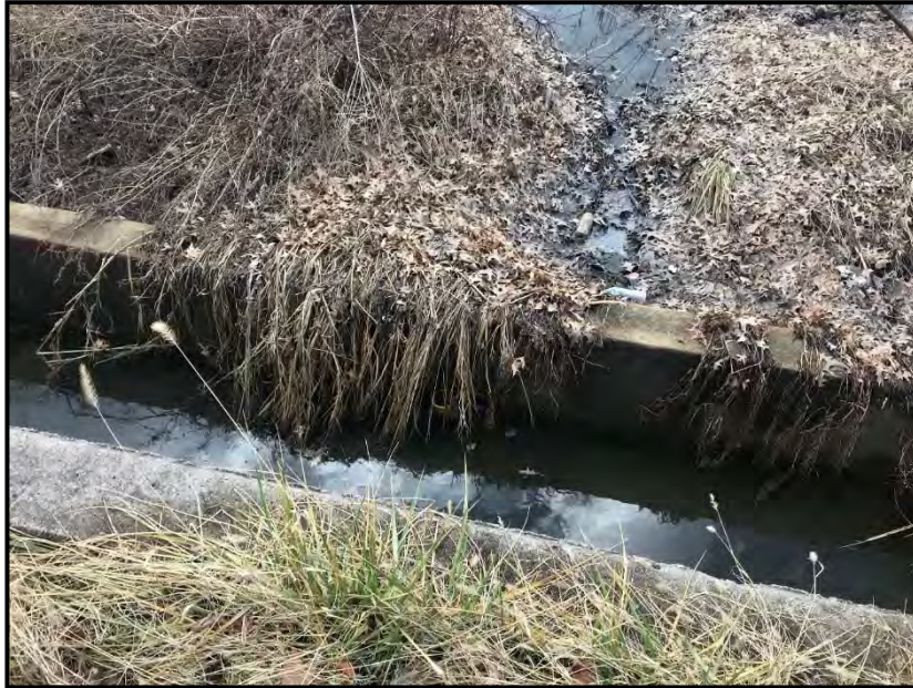
Figure 4-60: Outflow with standing water, assumed sedimentation within the low flow orifice
