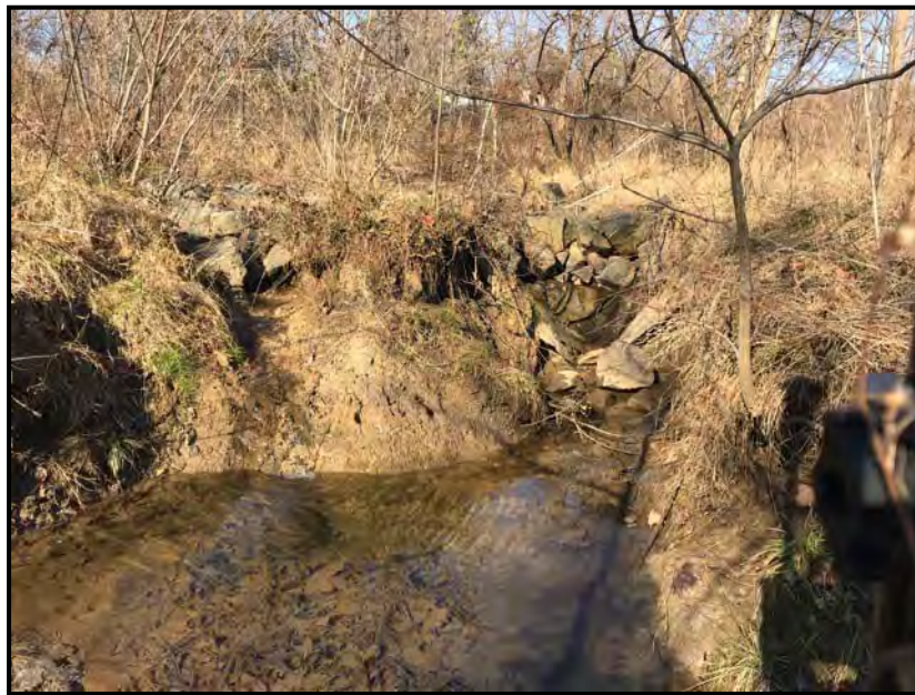
Figure 8-7: Erosion associated with culvert outfall.
