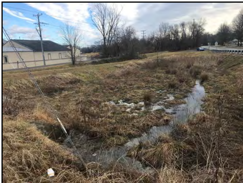
Figure 4-59: Continuous ponding at Dry Pond SWM24
