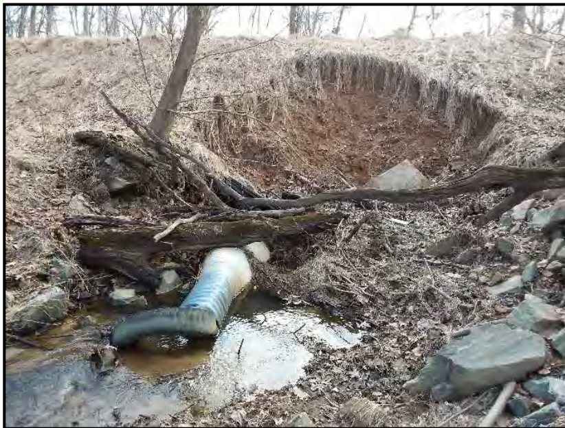
Figure 8-29: Collapsed culvert and eroded bank near Sleeter Lake
