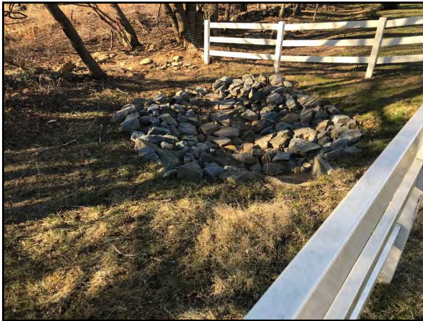
Figure 4-56: Erosion along outfall swale
