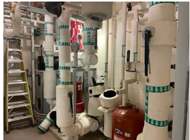
A geothermal exchange system at the Animal Shelter.
