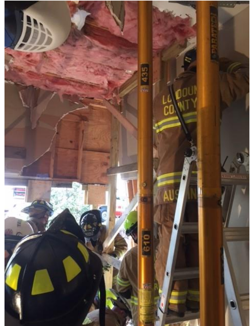
View of Pneumatic Shore Placement and Installation of Two-Piece Vertical Shores.
