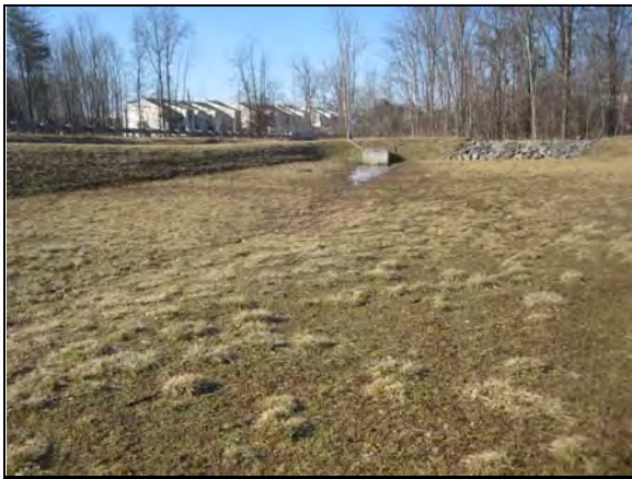
Existing stormwater detention facility, with a small amount of water pooled in front of dewatering structure
