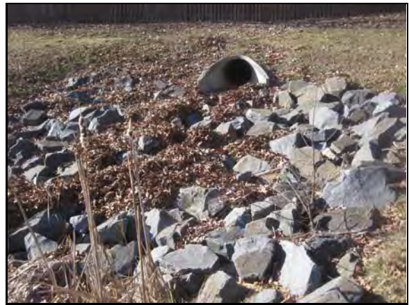
Pipe outfall that discharges to pond
