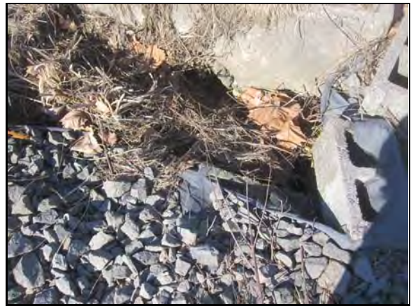
Damaged dewatering structure
