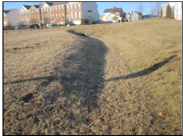
Existing drainage swales provide an excellent opportunity for conversion to bioswales
