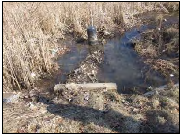
Dewatering structure clogged with sediment and debris
