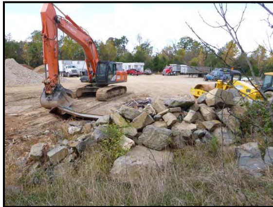
Figure 4-31: Outside Storage of Bulk Materials without the Benefit of Silt Fencing at HSI-008
