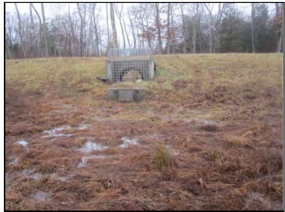
Control structure for existing dry pond
