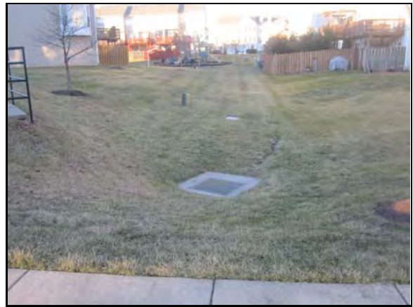
Swale between townhomes enters grate inlet before entering pond
