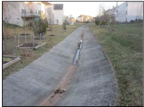
Concrete swale
