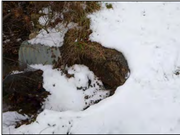
Headcut occurring beside pipe culvert
