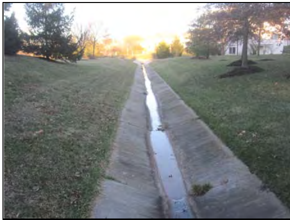
Concrete swale
