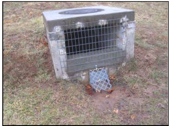
Dry pond control structure
