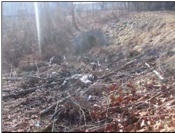
Outfall draining to dry pond; accumulated debris in foreground
