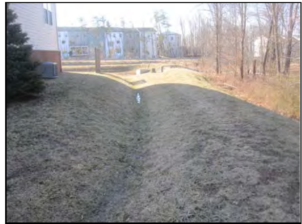
Grass swale leading between townhomes to the stormwater pond
