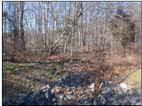
Channel downstream of pond is in stable condition and has little erosion
