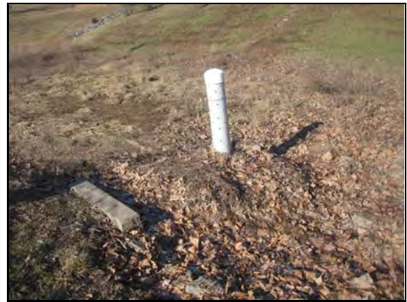
Stormwater pond dewatering structure
