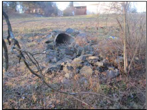
Pipe outfall draining to pond
