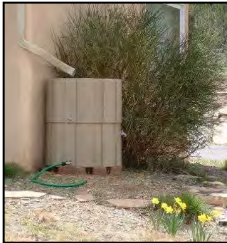
Figure 5-8: Rain Barrel Standard Section and Photos of Rain Barrel and Above-ground Cistern (Sources: Prince George's County 1999; www.aridsolutions.com ; and www.plastmo.com )
