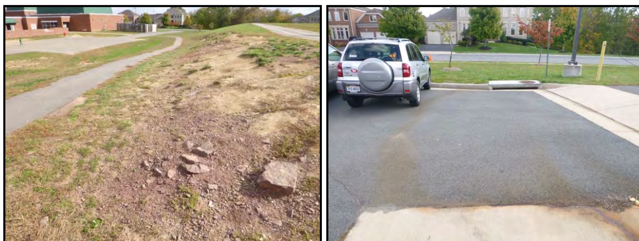
Figure 7-5: Terracing Opportunity to Address Erosion (left) and Stains Leading from Dumpster to Storm Drain Inlet (right) at ISI-004
