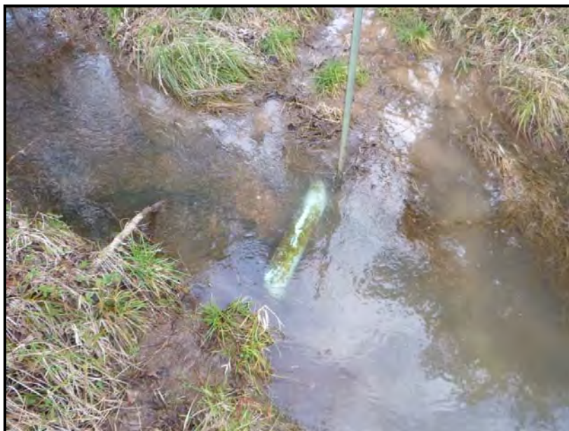
Figure 4-14: Exposed Pipe within the Streambed of Upper Broad Run
