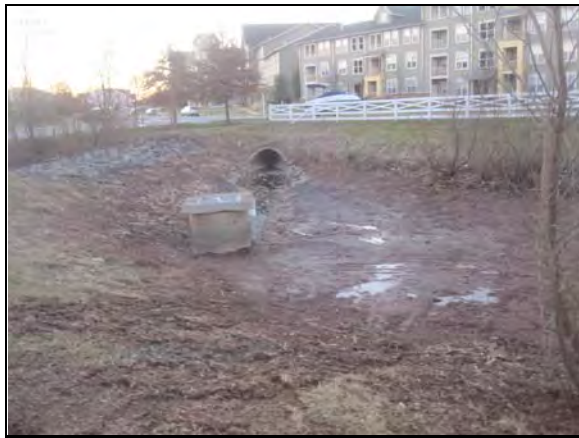
Pipe outfall enters pond directly in front of dewatering structure
