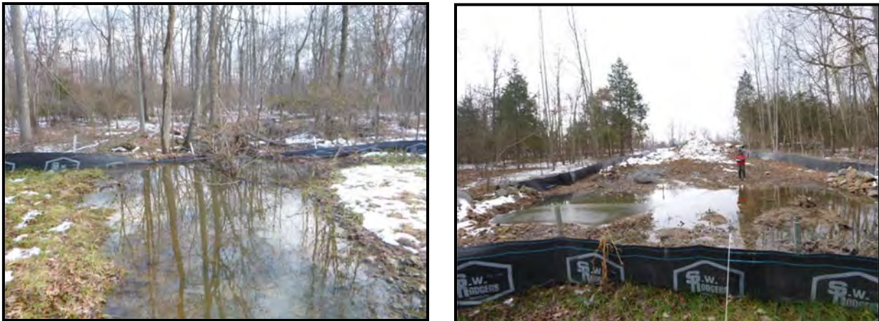
Figure 4-9: Near Stream Construction with Super Silt Fence Placed within the Stream in an Area with a Recently Installed Sewer Line, Rated in the Survey as Severe (Left Photo) and Absence of Super Silt Fencing Along Right Bank is Exposing Stream to Runoff from Active Construction Site Rated in the Survey as Severe (Right Photo).
