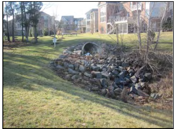
One of the many pipe outfalls that discharge to the wet pond
