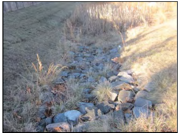
Riprapped swale leading to pond
