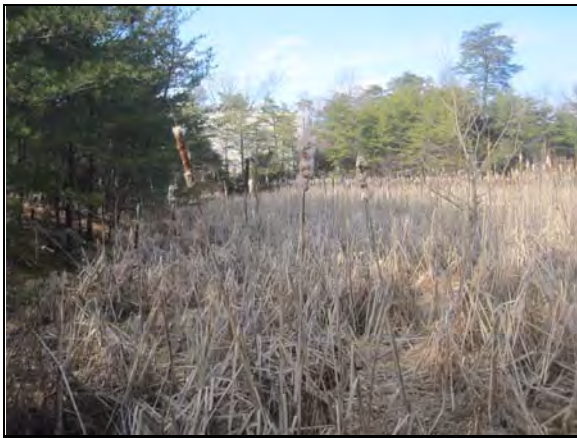
Stormwater pond currently filled in with cattails
