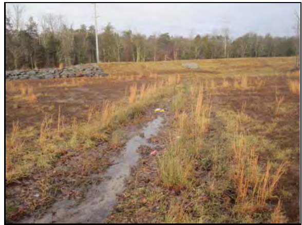
Flow path being created between outfall and dewatering structure
