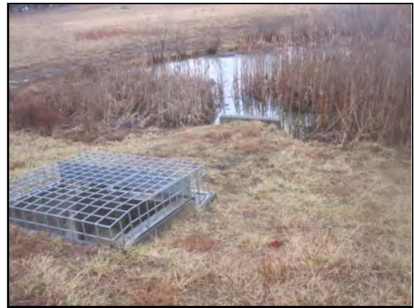
Dewatering structure for existing stormwater pond
