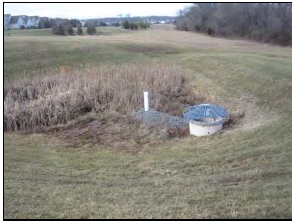
Existing extended detention dry pond
