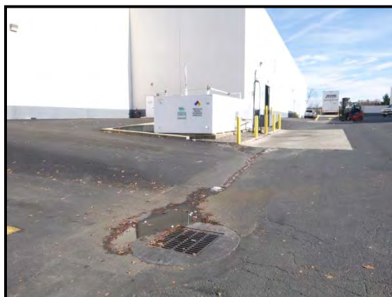
Figure 4-30: Uncovered Fueling Station at HSI-014. Note that the liquid near the storm drain inlet is melted snow.
