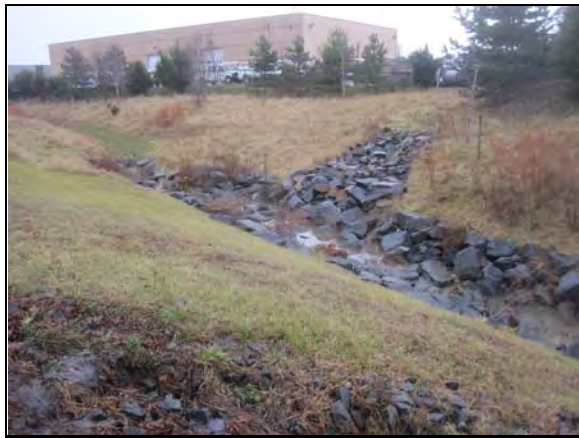
Riprapped channel from parking lot to pond where a bioswale is recommended
