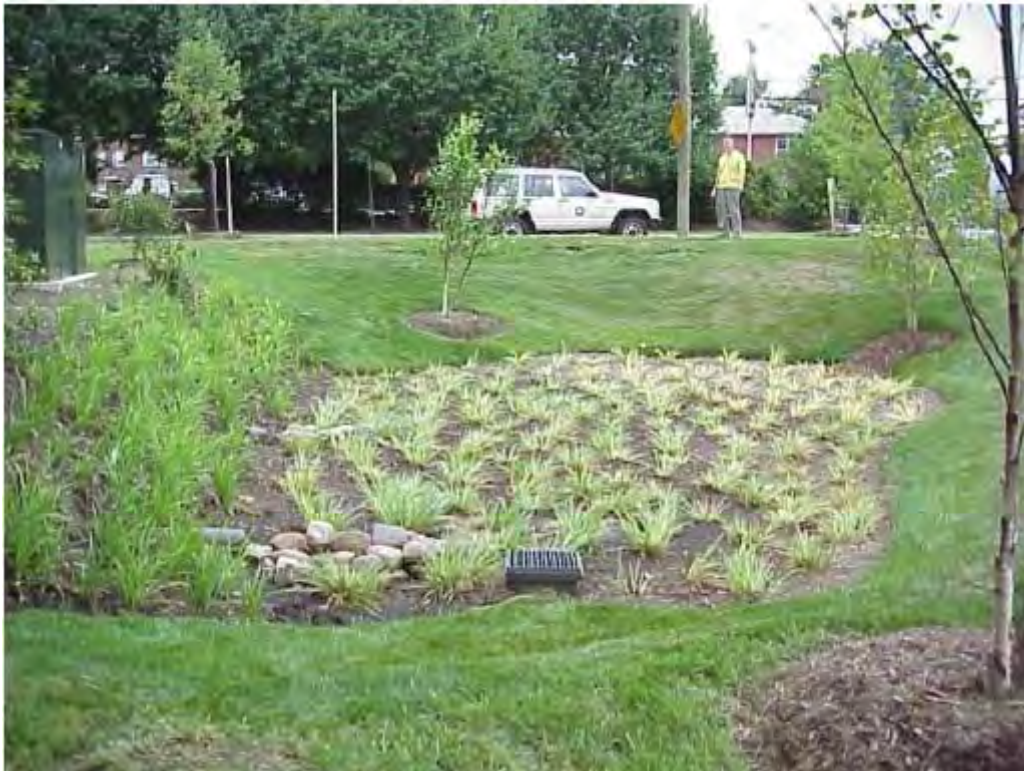
Figure 5-4: Photo of Bioretention Draining a Rooftop at a Commercial Facility (Virginia DEQ 2011c)
