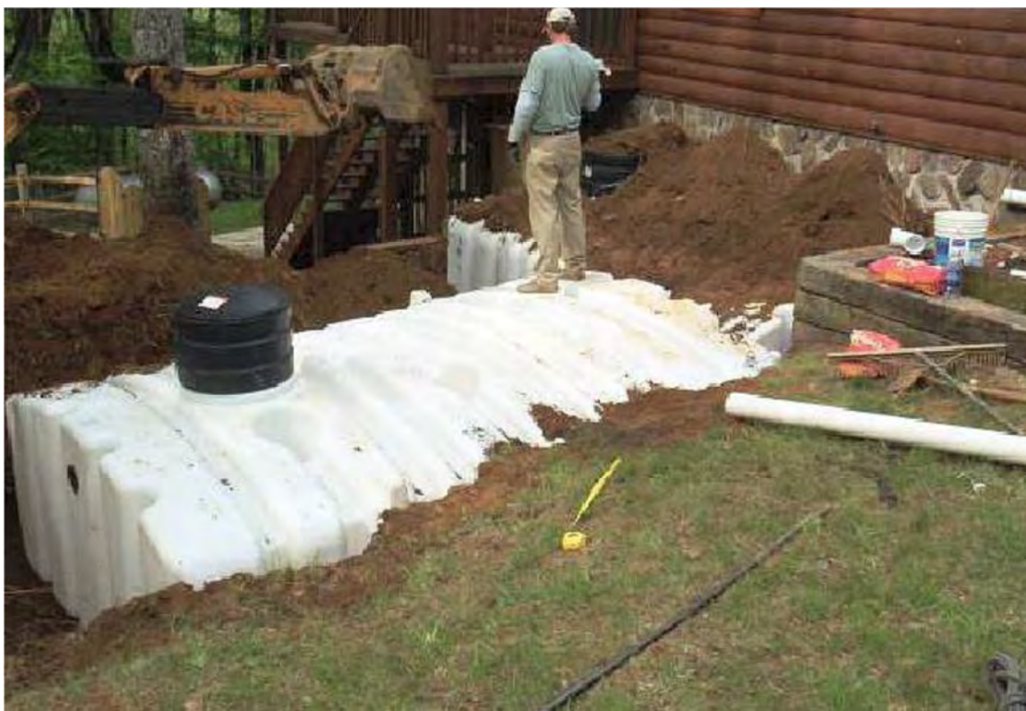
Figure 5-9: Subterranean Cistern (Virginia DEQ 2011f)
