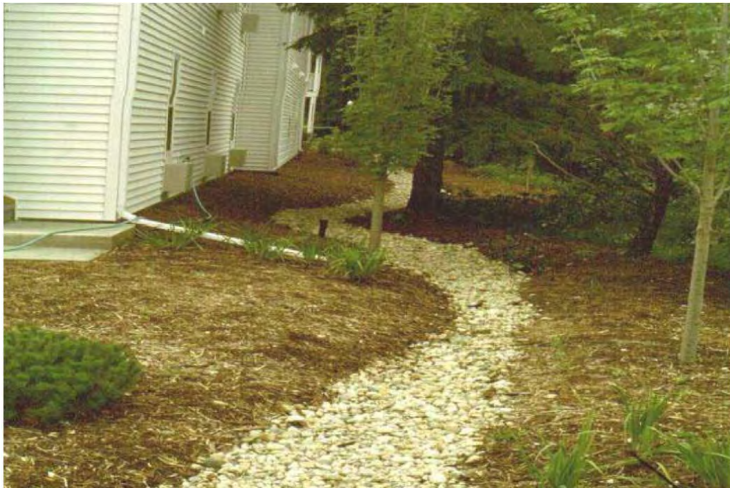
Figure 5-2: Residential Infiltration Trench (Virginia DEQ 2011b)
