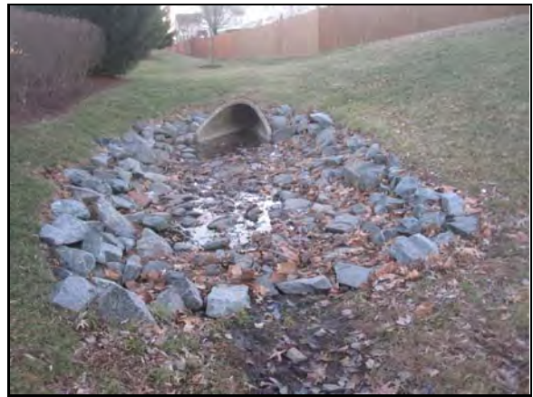
Riprapped pipe outfall entering pond
