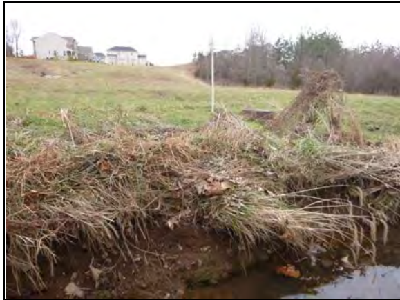
Bank erosion near sewer crossing, unforested riparian
