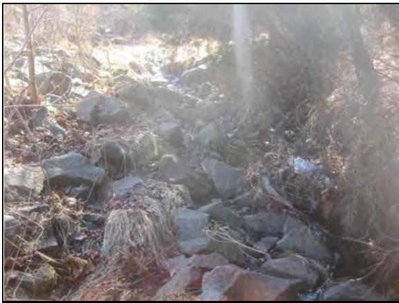
Riprapped flow path to pond that may be converted to a step pool conveyance
