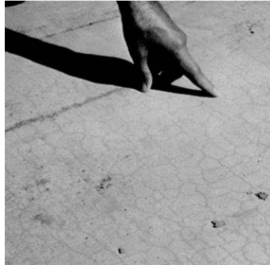
Crazing Crack
