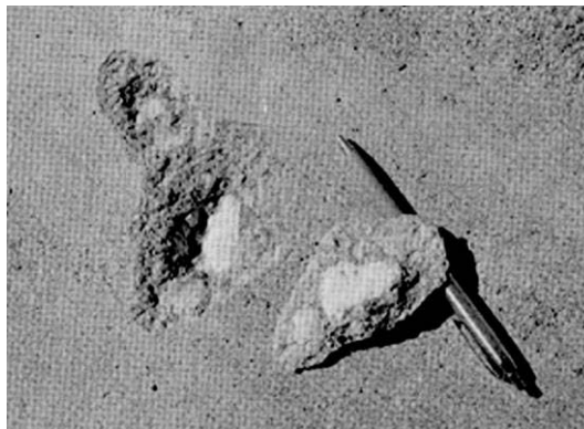
A popout is a small fragment of concrete surface that has broken away due to internal pressure, leaving a shallow, typically conical, depression.
