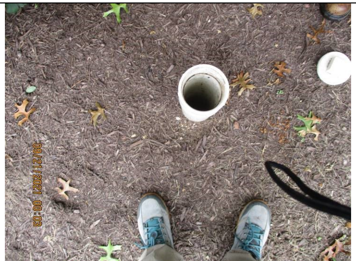
No. 12 – Clean-Out/Observation port connected to the base of the Bioretention Basin.
