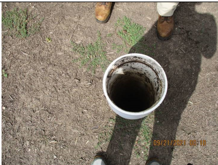
No. 11 – Bioretention Overflow (Connected to the Media).
