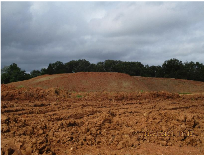
Fig. 3 Description: Stock pile needs stabilization.
