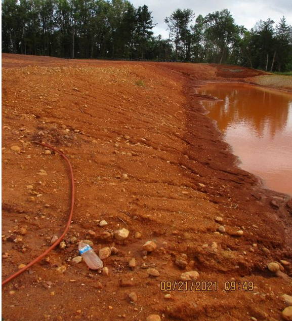
Fig. 3 Description: Stock pile needs stabilization.
