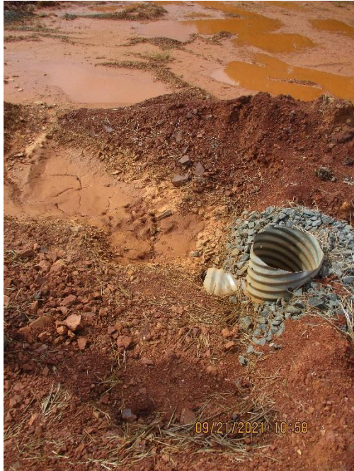
Fig. 7 Description: Slope to the left of SW channel if figure 6- needs stabilization
