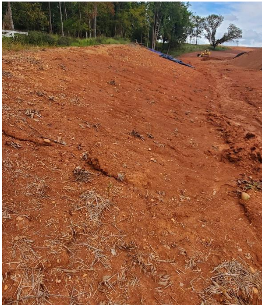
Fig. 7 Description: Slope to the left of SW channel if figure 6- needs stabilization
