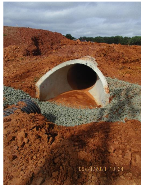
Fig. 8 Description: Sediment observed in SW pipe
