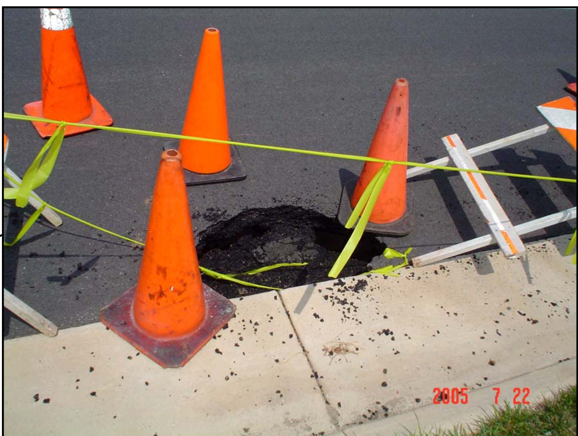
Route 15 Business near Dry Hollow Road (photograph date: July 22, 2005) Sinkhole is approximately 3 feet in diameter and 6 to 8 feet in depth.
