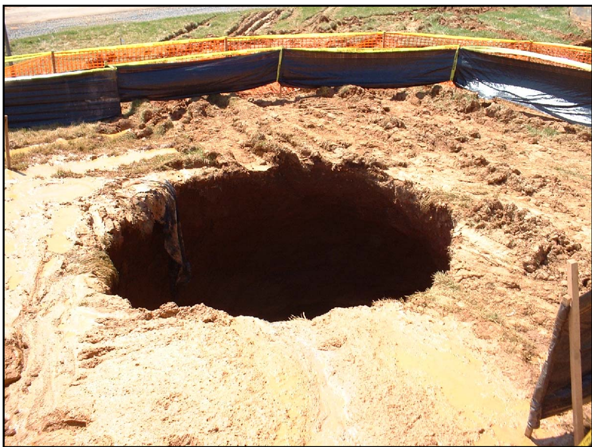
Leesburg Crossing Subdivision (photograph date: April 6, 2005) The sinkhole is approximately 6 feet in diameter and opened during well installation.
