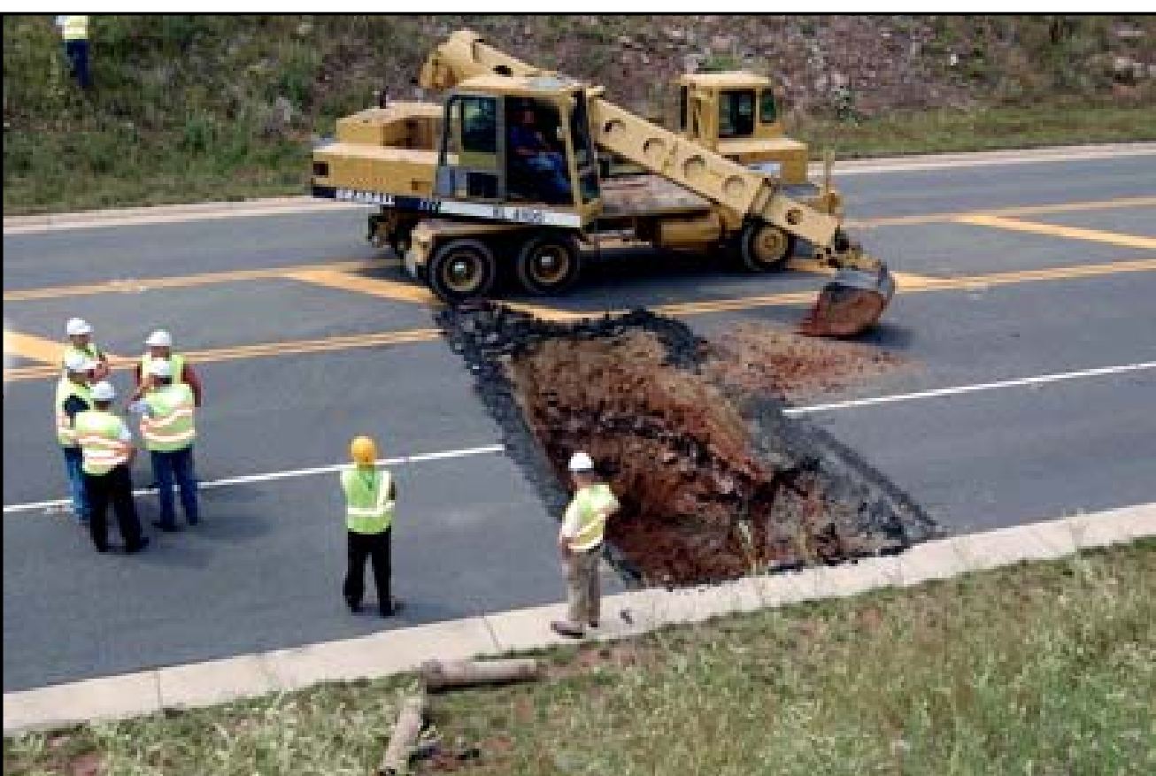
Approximately one year later, the sinkhole reopened at the same location. The sinkhole is approximately 20 feet in diameter and 15 to 18 feet in depth. (photograph date: June 28, 2006; source: Leesburg Today)
